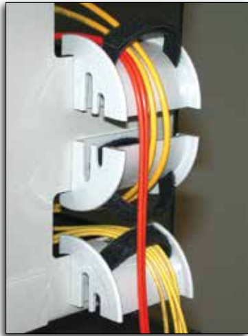
Patch Panel Egress
